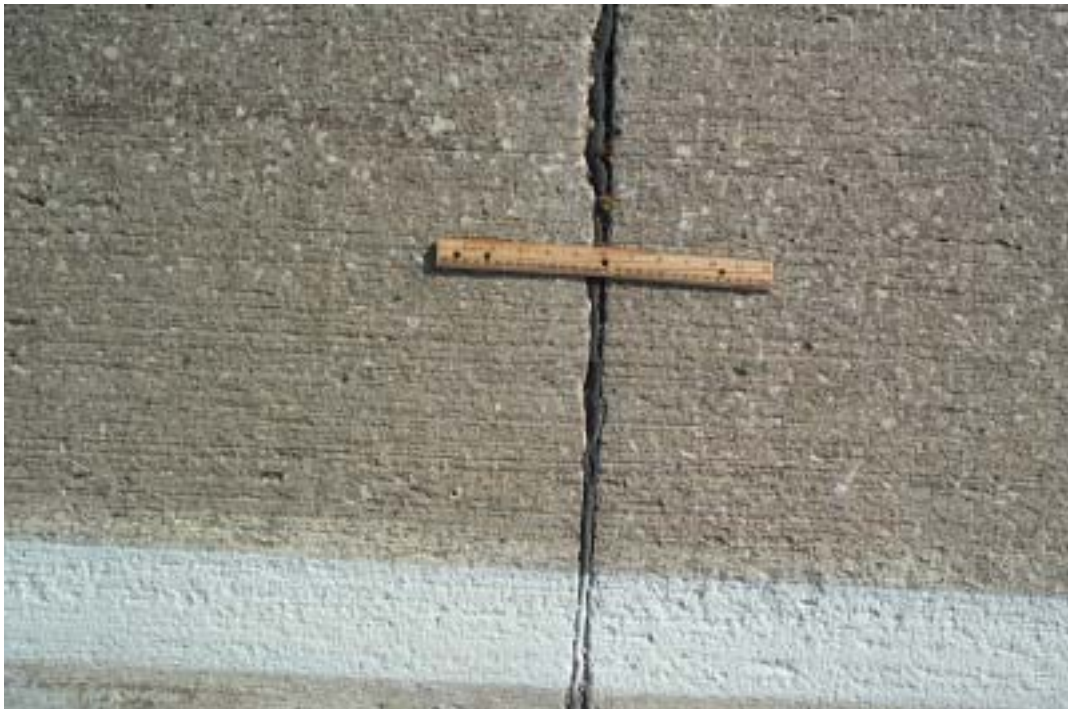
Figure C.12. Light turf drag section.
