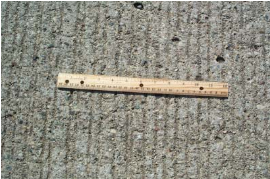
Figure C.10. Transversely tined section.
